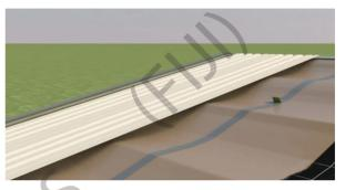
Use a plastic squeegee or blade to apply appropriate pressure to the tape. End joins should be overlapped by 600 mm if not taped.
